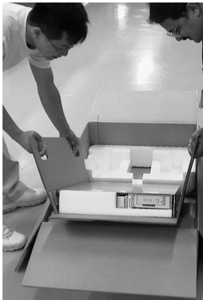
Figure 258. Slide the 2145 UPS to the edge of the carton
