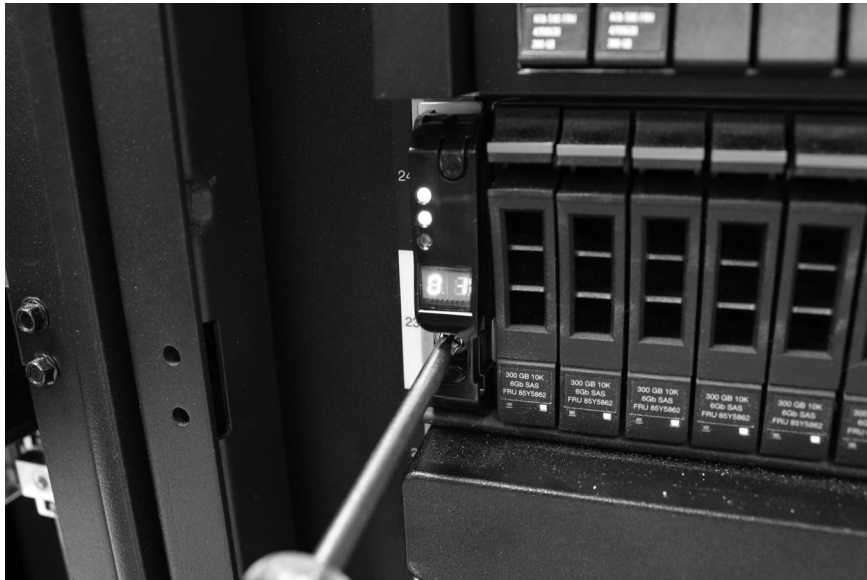
Figure 13. Securing an enclosure to a rack cabinet
