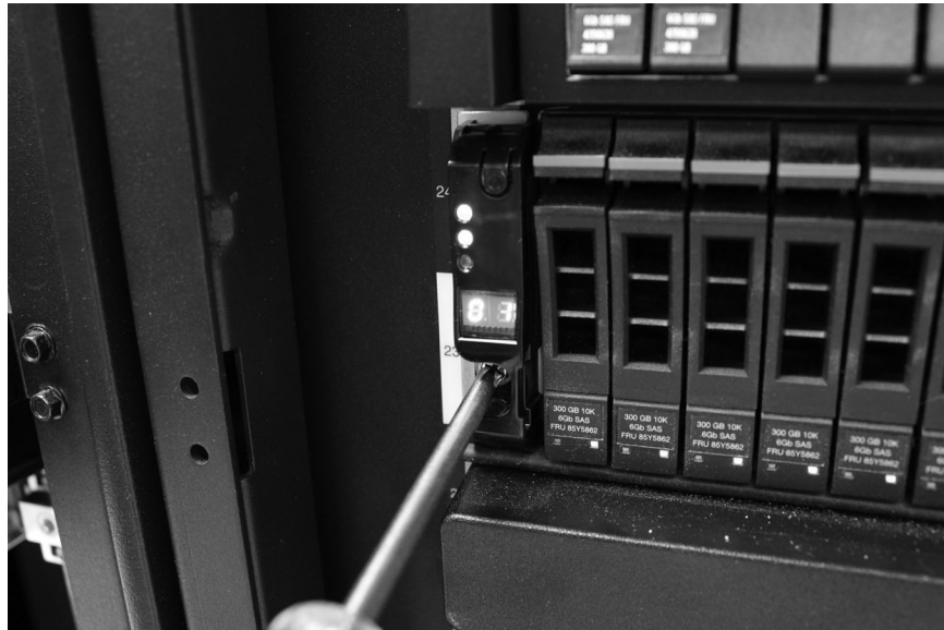
Figure 18. Securing an enclosure to a rack cabinet
