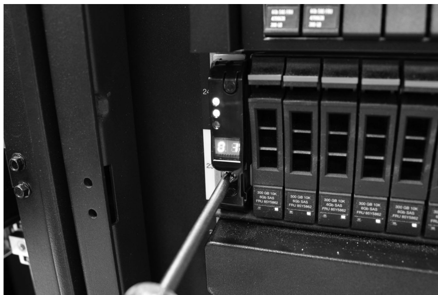
Figure 19. Securing an enclosure to a rack cabinet
