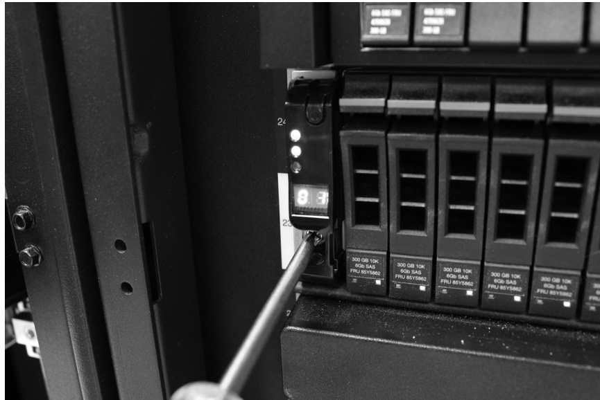
Figure 27. Securing an enclosure to a rack cabinet
