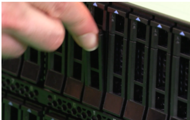
Figure 74. Completing the drive installation
