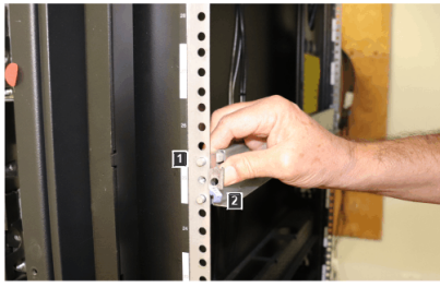
Figure 29. Installing the front rail bracket
